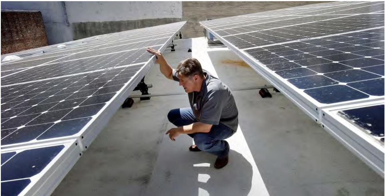
Figure 5. Ted van der Linden, Sustainability Director at DPR Construction, inspecting the PV array on the roof of their newly renovated San Francisco headquarters building. The building has submitted its LEED v4 Platinum certification to the U.S. Green Building Council as well as Net Positive Certified from the International Living Future Institute.
