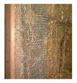
Figure 16: Facing Reinforcement
