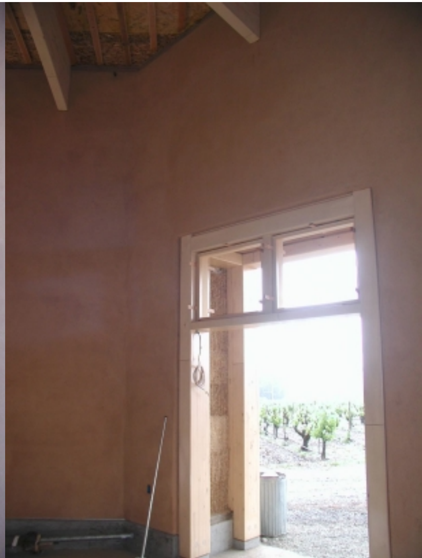
Site 4 – Interior View
