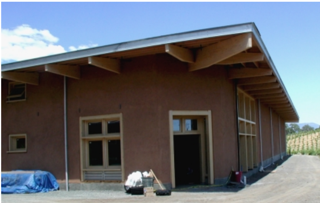
Figure 2.1: View of south-west corner at entrance door
