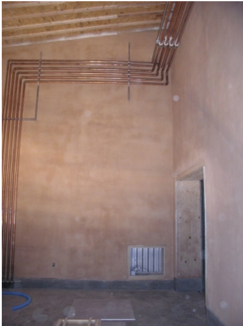
Site 2 – Interior View
