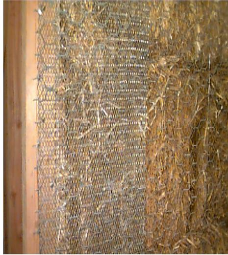
Figure 16: Facing Reinforcement
