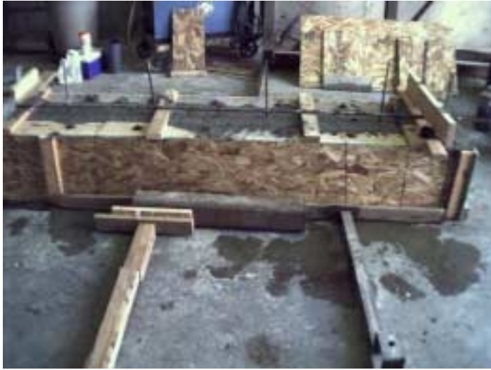
Figure 2 – Side view of poured footing
