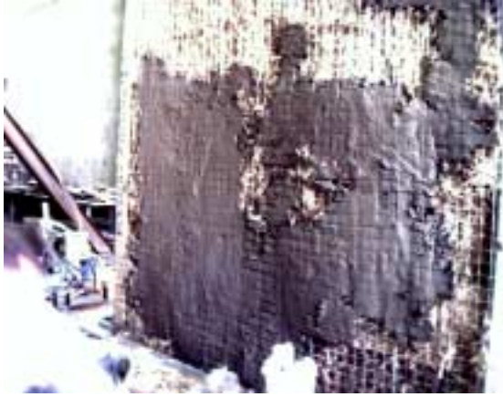
Figure 8 – Partial scratch coat applied
