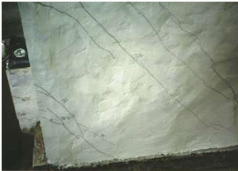
Figure 15b – Outer shear cracks in right face
