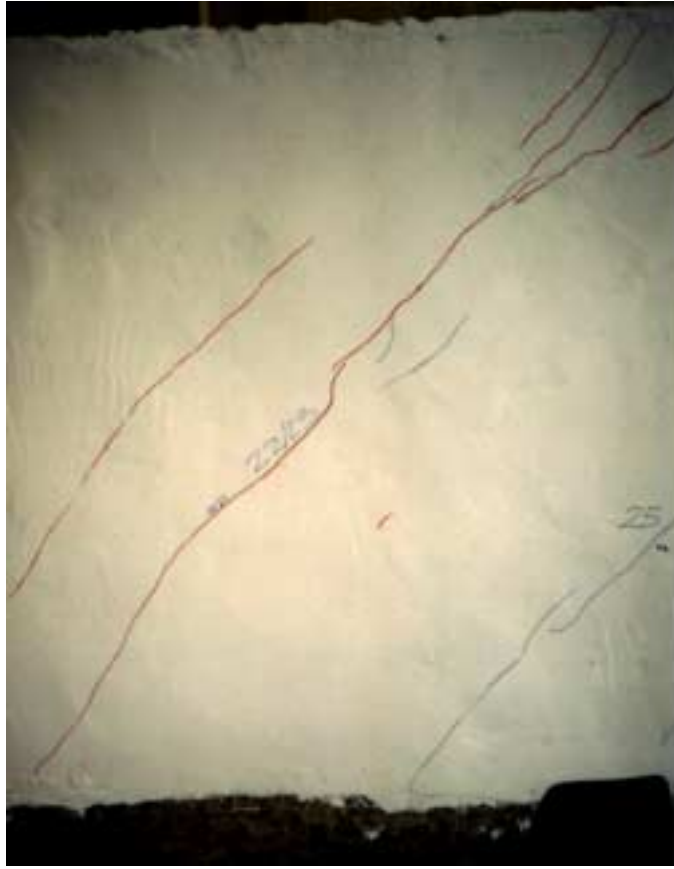
Figure 11 – Cracked left face after tests 1 & 2
