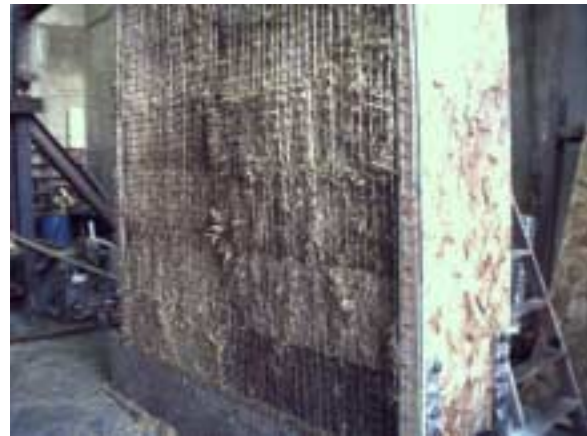
Figure 5 – Mesh over bales
