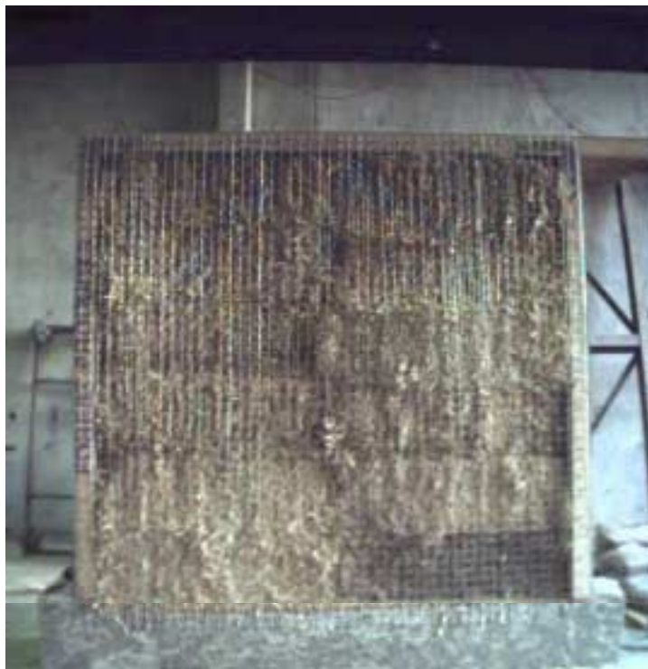
Figure 7 – Unplastered wall elevation
