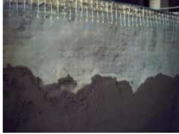
Figure 9 – Partial brown coat applied
